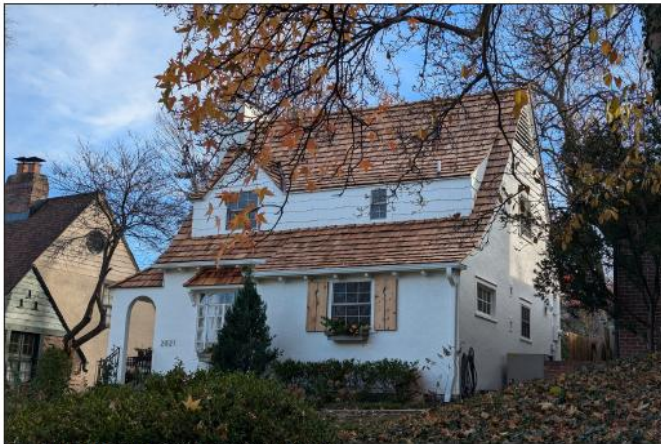
2. Primary (north) and west elevations, View SE Part 2 Scope Item #2: new roof
